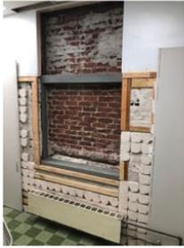
Before: Removed brick from previously closed up window
