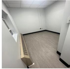
After: Removed tiles and installed drywall, new flooring, fresh paint, and ceiling grid/ lighting
